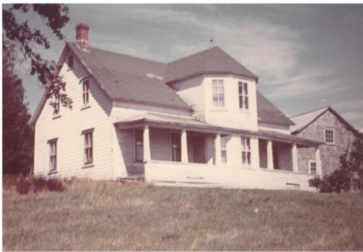
*"...someone did paint the house and shingled the roof with Arrow-lock asphalt shingles. I helped put on quite a number of them. Cost in 1938 was app. \$2.60 per square (10" x 10")...Note the piazza roof is covered with corrugated galvanized roofing, quite likely over the wood shingles. A common thing for that period. This picture was taken after haying time and the mowing leaves something to be desired. Note the streaks of dried hay left by the mowing machine." Grandpa was quite particular*
